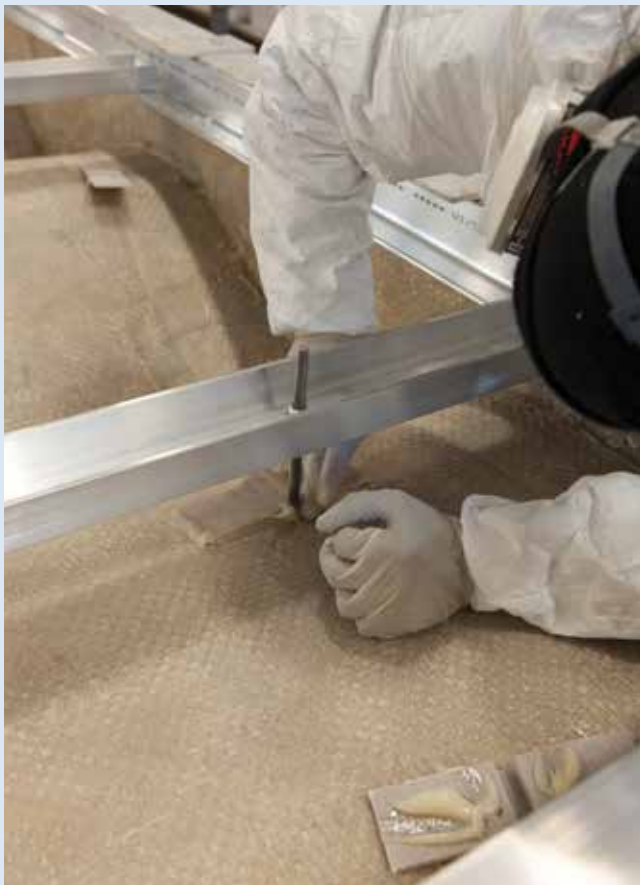
5 Attachment plates for aluminum framing were then bonded to the FRP, enabling aluminum stiffening ribs to be mechanically fastened down the length of each panel.
